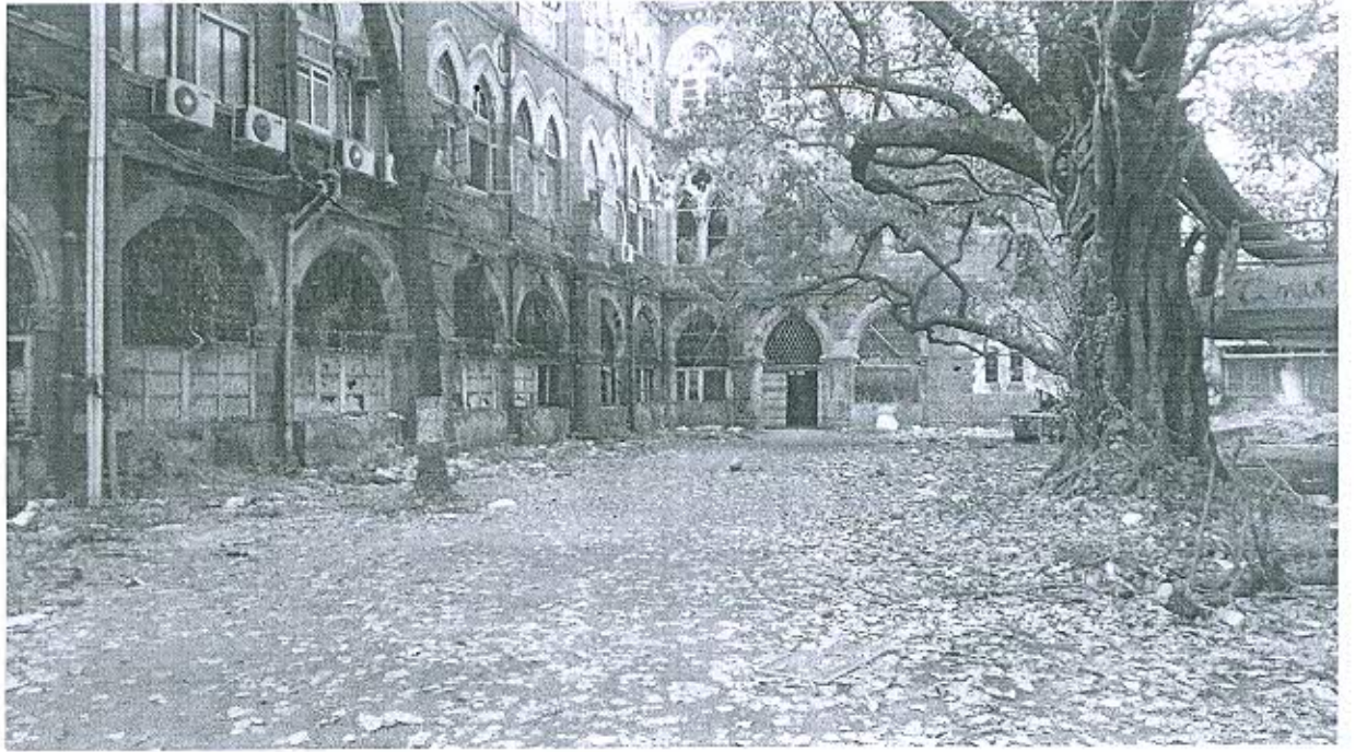
Rear view of the building
