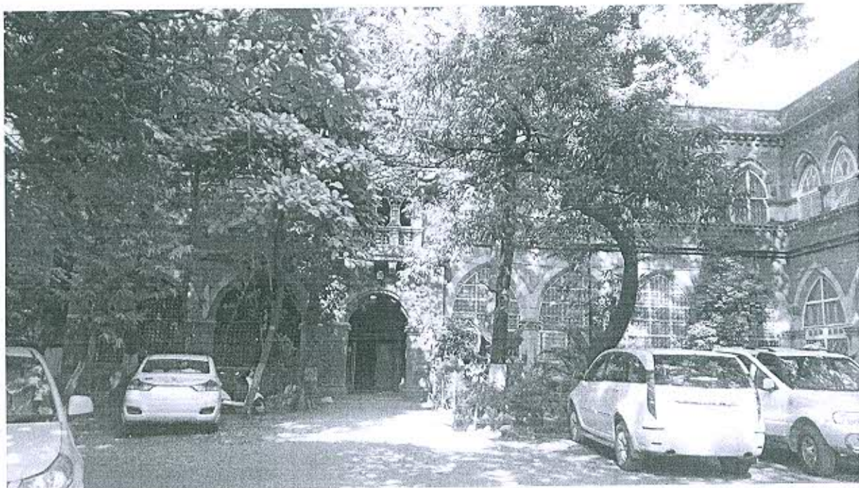
Front view of the Building
